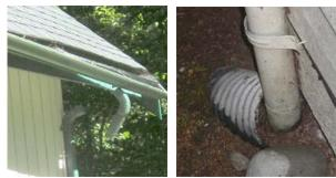
Gutter mounts failing and the downspout is disconnected. Keep downspout drains clear of mulch and debris.
