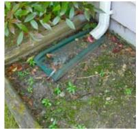
This splash block is discharging in a planter. Water trapped next to the building may end up under the home.
