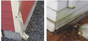
Repair any crushed or incomplete drains assuring they discharge away from the home.
