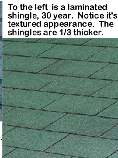
On the right is a standard 3 tab roof. Thinner material. Average life span 15 years.
