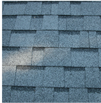
On the right is a standard 3 tab roof. Thinner material. Average life span 15 years.
