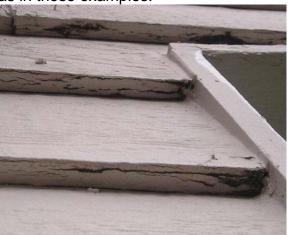
The bottom edge of LP lap siding is where the failure is first evident.
