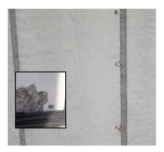
Sheet LP fails in the grooves, nail holes and penetrations.
