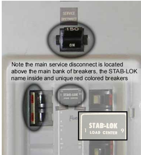
Unique main location (not all FPE equipment will have this main breaker), red colored breakers and STAB-LOK name inside
