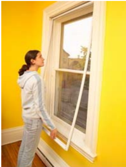
Adding interior magnetic window coverings will save energy and are easy to install
