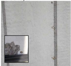
This type fails in the groves nail holes and penetrations.
